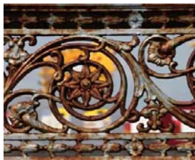
Clean, prime and paint historical metal work
