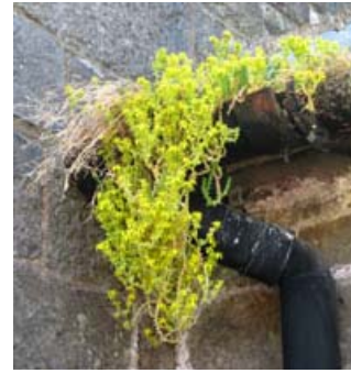
Clear gutters, downpipes and hoppers
