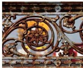
Clean, prime and paint historical metal work
